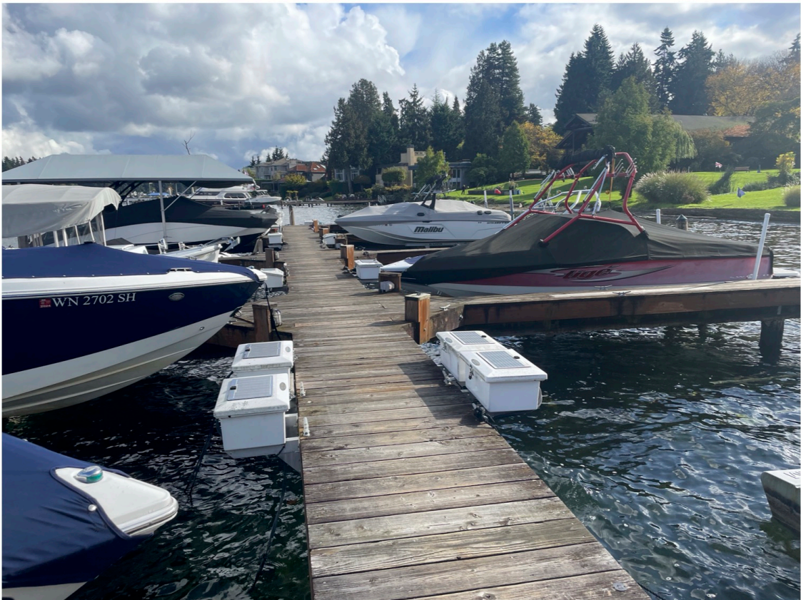
Photo 2 - Existing pier looking east from main dock.
