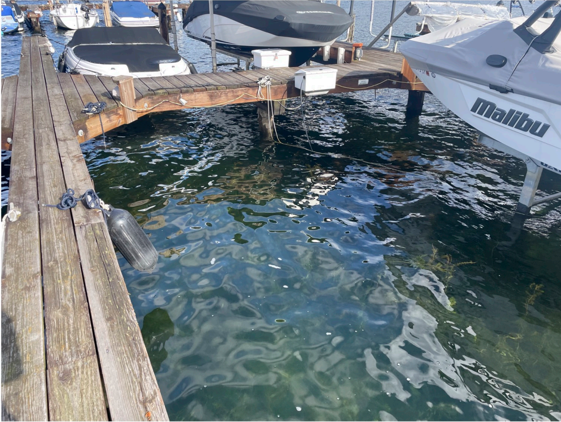
Photo 5 - Existing slip looking waterward.
